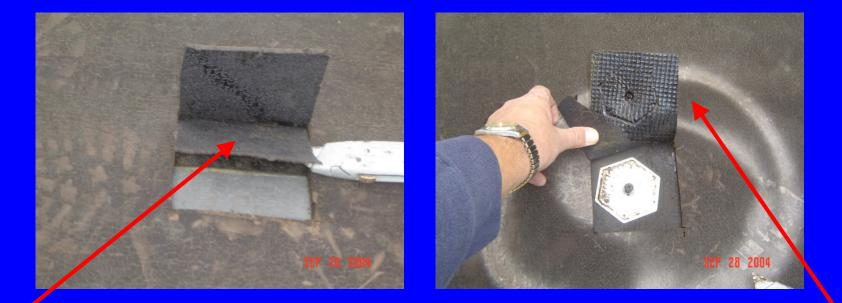
Here the contractor did not install a cover board insulation, adhere the base sheet to the insulation and did not even melt the torch applied modified bitumen membrane. This roof flaps in the wind.
